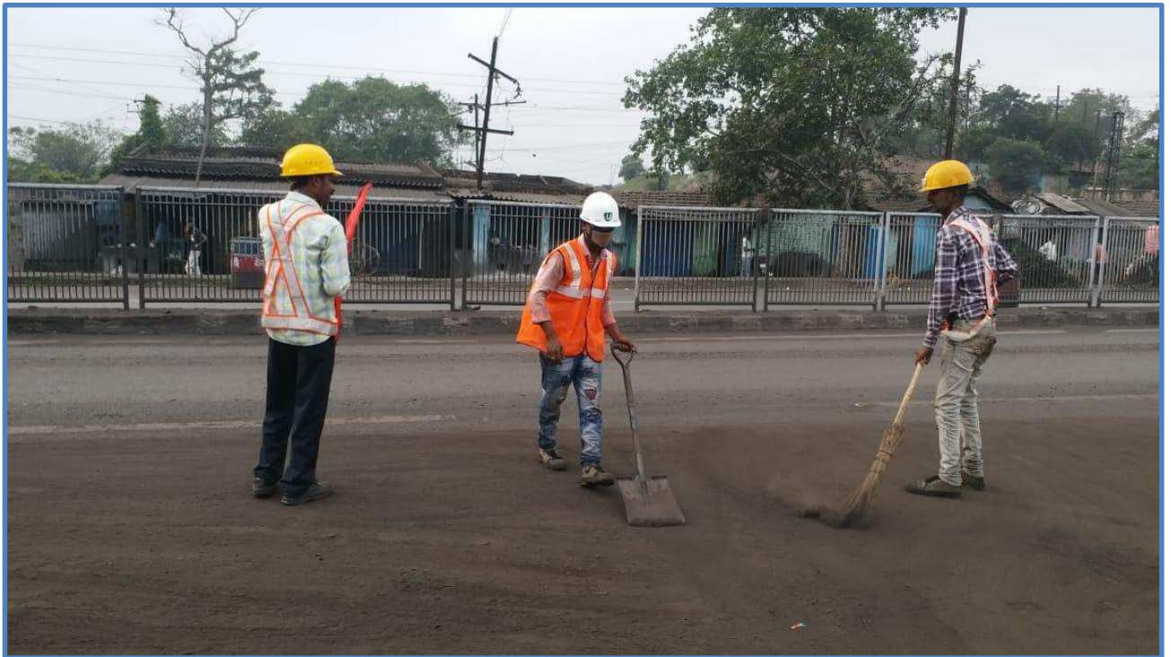
Picture 3 – Manual Sweeping of Public Road
