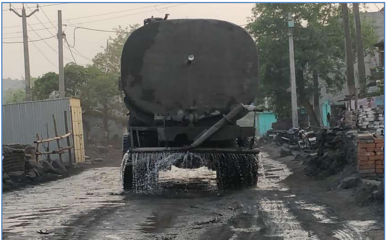
Picture 2 – Water Sprinkling on Transportation Road
